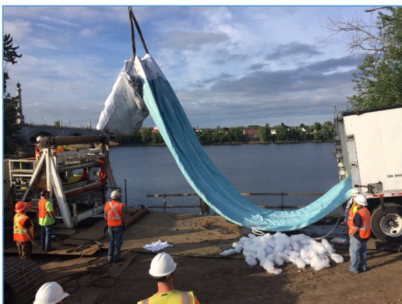
Prefabricated fiberglass liner insertion – fall 2018
