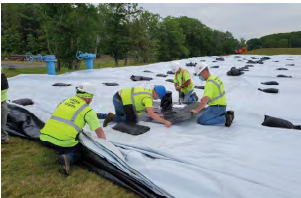
Top: The Process Control Manager consults with the Half-Plant Coagulation Trial contractor at West Parish Filters. Bottom: A temporary tarp is placed over the clearwell to limit leaks through the existing concrete roof structure.
