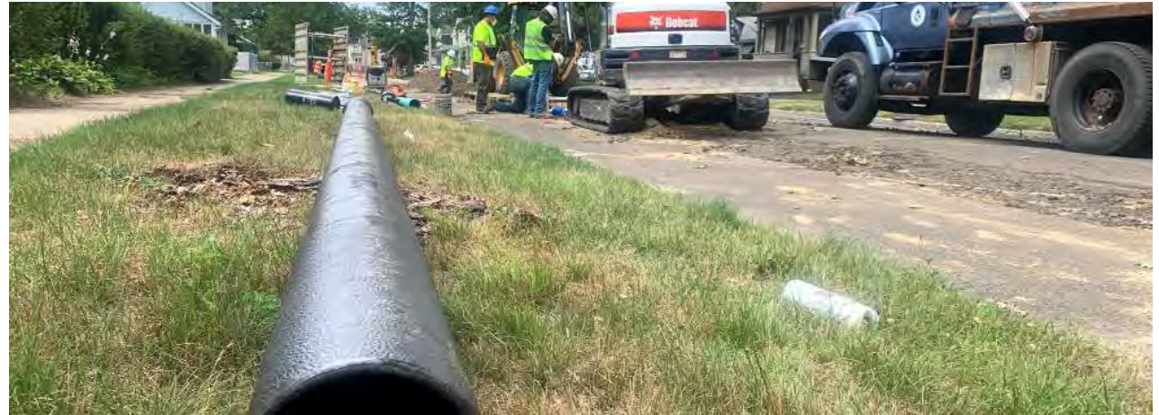
Above: Water main is replaced on Farnsworth Street. Opposite page, top: A crew inspects the diversion gates at Cobble Mountain Reservoir; Bottom: An aerial view of slow sand manholes and blue DigSafe paint in preparation for construction of the new clearwell.
