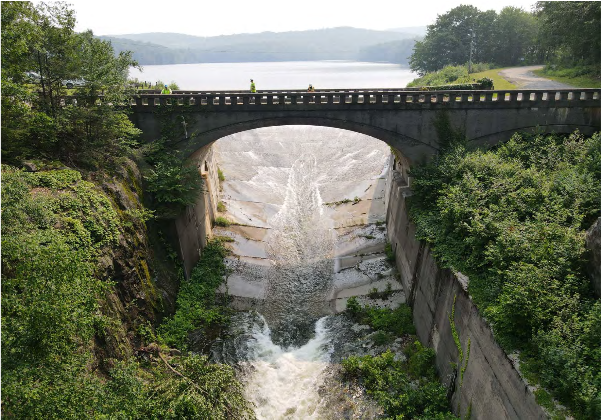
Above: The Cobble Mountain Reservoir spillway.
