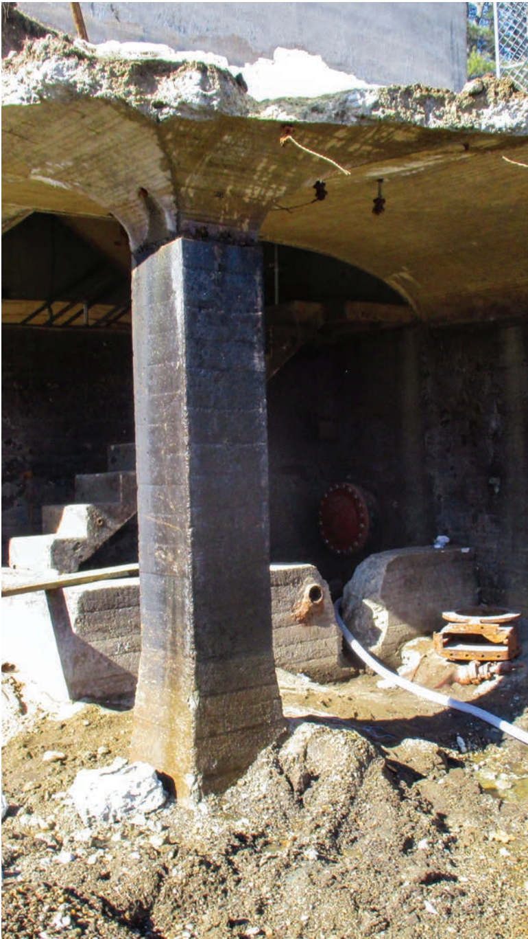
At left, a slow sand filter is exposed to sunlight for the first time since 1909 as it is demolished in early 2021 to create the site for the new Clearwell and Backwash Pump Station project (right).
