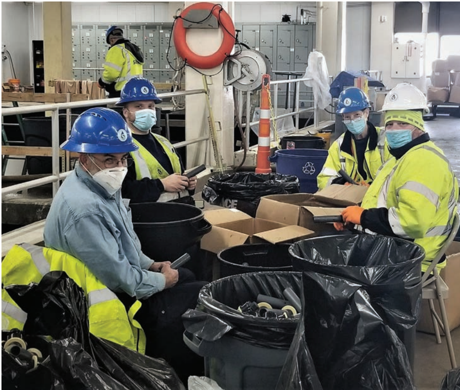
Above: Water Operations staff work on cleaning and replacing nozzles on the other non-damaged rapid sand filters.
