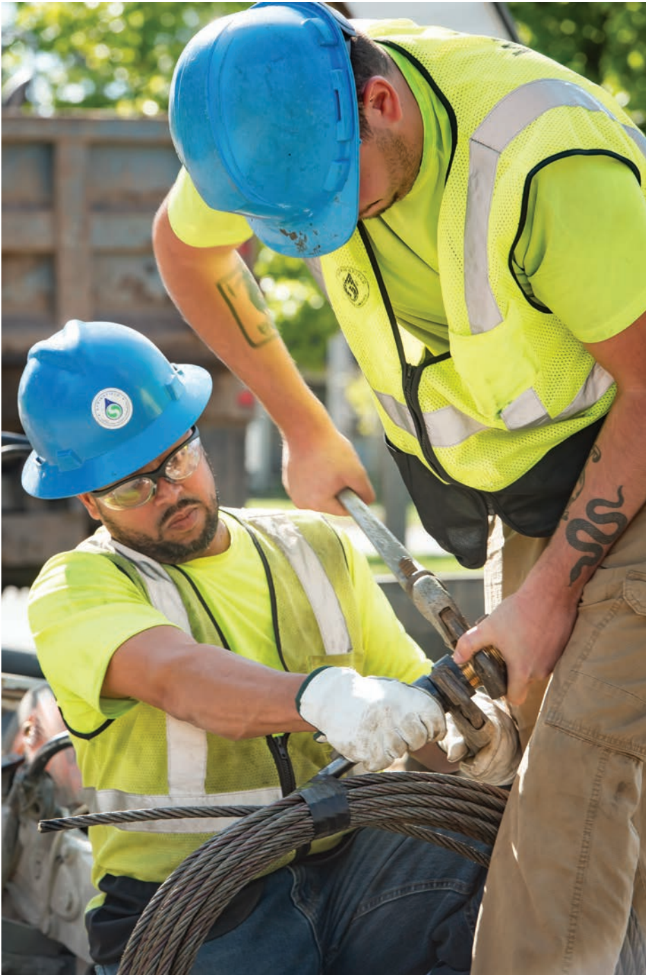
Commission crews prepare equipment for a distribution system upgrade.
