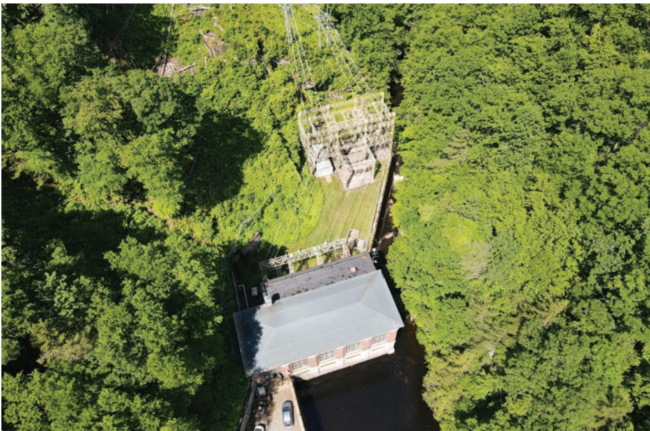
An aerial view of the Cobble Mountain Hydropower Plant.
