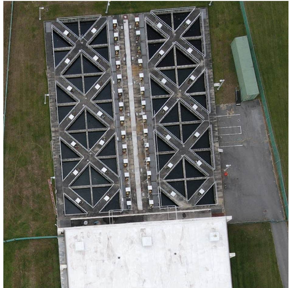
The chemical room supports the functioning of the existing flocculators at West Parish Filters, shown above. The flocculators mix coagulants that bind to dissolved solids in the raw water, facilitating their removal during filtration.
