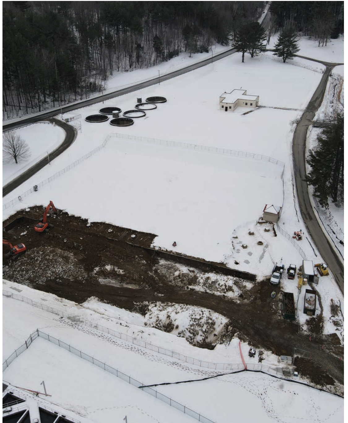
At left, a slow sand filter is exposed to sunlight for the first time since 1909 as it is demolished in early 2021 to create the site for the new Clearwell and Backwash Pump Station project (right).
