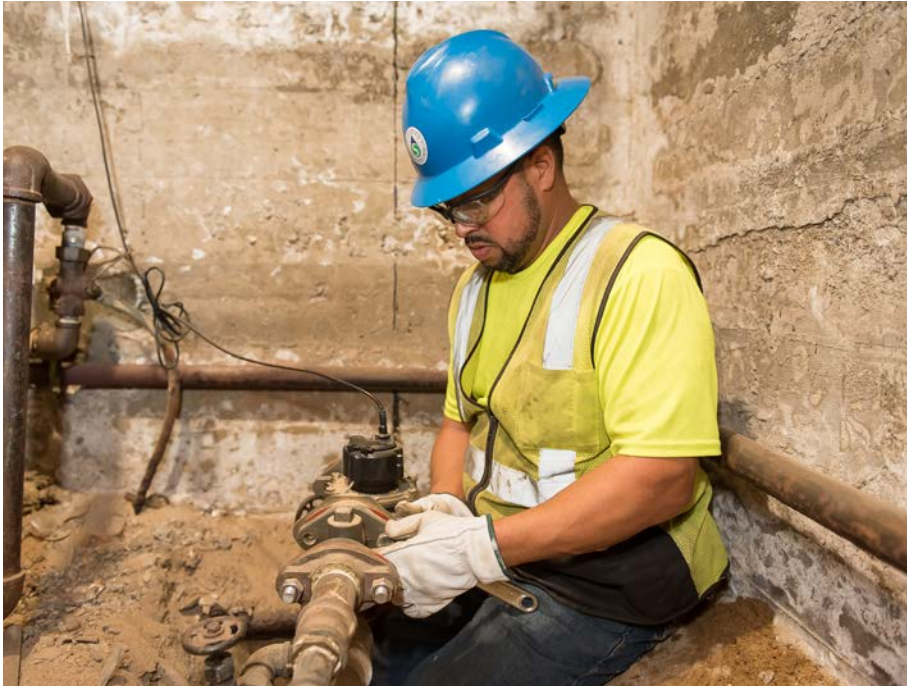
A Field Services crew member changes a water meter at a customer's property.
