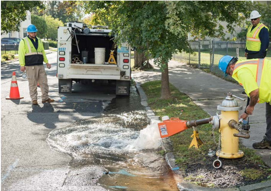
The Commission regularly flushes its distribution system to address water age and clear pipes of sediment.
