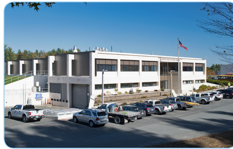
West Parish Filters Water Treatment Plant in Westfield
