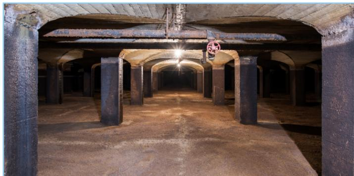
Pictured above is a 1920s-era slow sand filter, still in use today to meet peak demand. All slow sand filters will be eliminated upon construction of the new treatment plant.
