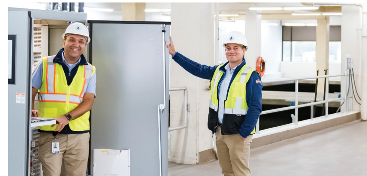
Information Technology staff maintain the Commission's technology infrastructure, including West Parish Filters Water Treatment Plant operating systems.
