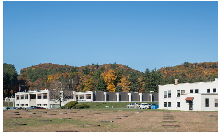
West Parish Filters Water Treatment Plant in Westfield
