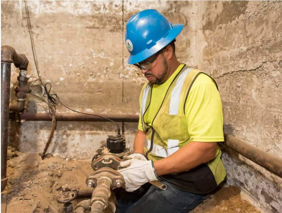
A Field Services crew member changes a water meter at a customer's property.
