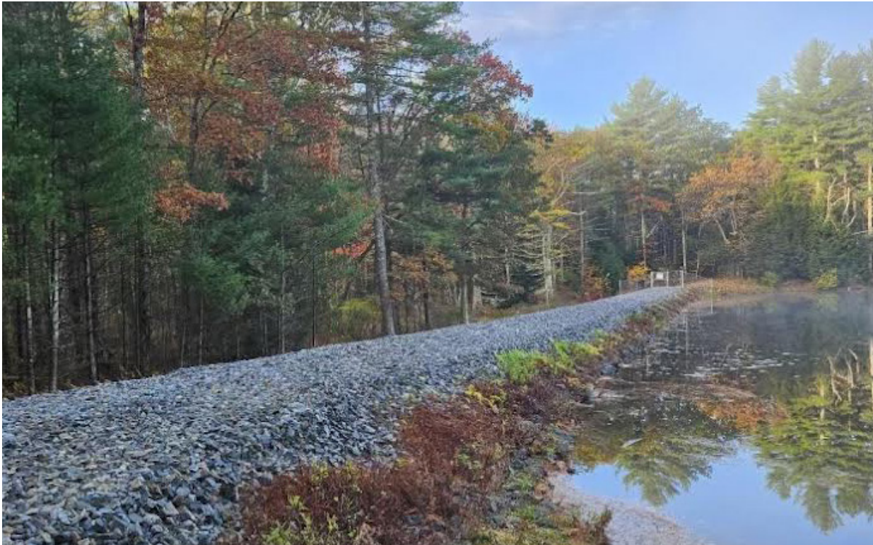
Additional stone was added to Knight's Pond Spillway to allow for easier public access and travel.
