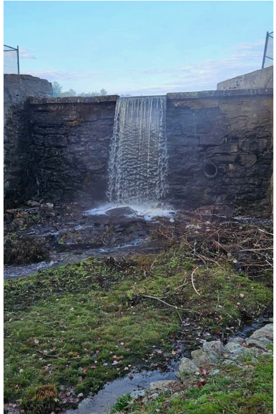
Knight's Pond Dam Spillway.
