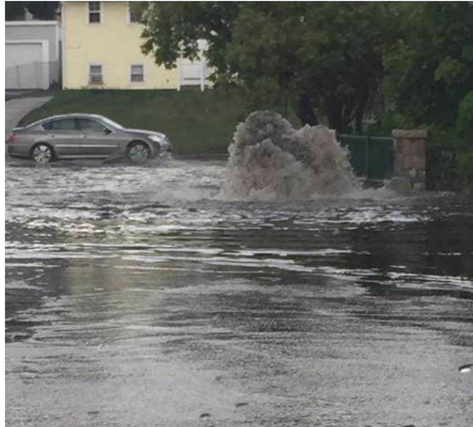
An overflowing sewer manhole on Mill Street, just upstream of the siphon
