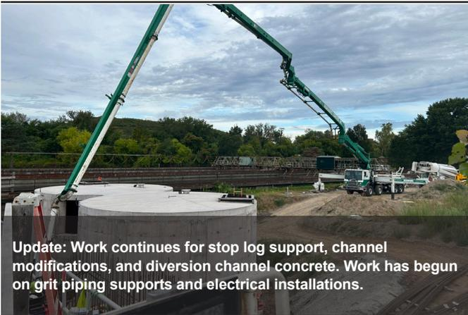
Update: Work continues for stop log support, channel modifications, and diversion channel concrete. Work has begun on grit piping supports and electrical installations.
