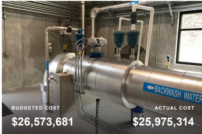
The WPF clearwell and backwash pumps replacement project replaced the underground clearwell structure from the 1920s and installed new backwash pumps at the treatment plant. This has improved water quality, energy efficiency and increased the system redundancy.
