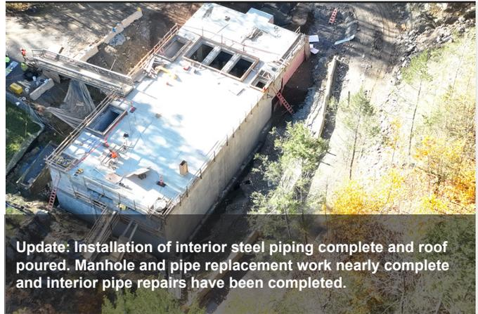
Update: Installation of interior steel piping complete and roof poured. Manhole and pipe replacement work nearly complete and interior pipe repairs have been completed.
