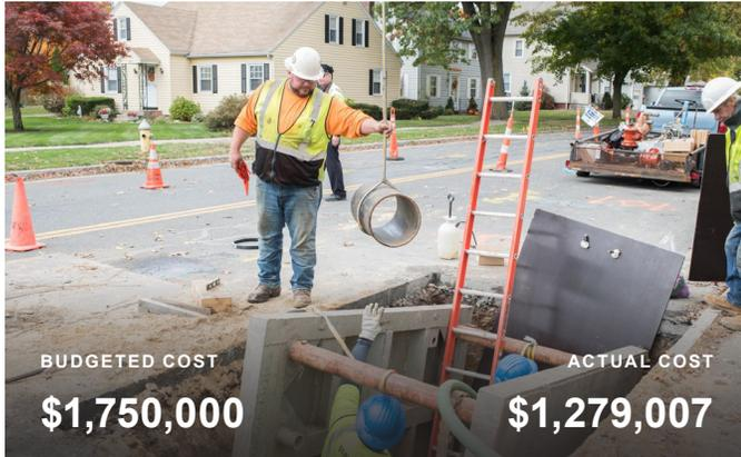
The FY2022 Water Distribution Improvements Project was constructed to replace watermain on Massachusetts Avenue and Narragansett Street with new 8" and 6" ductile iron class 52 pipe. This work replaced approximately 3,600 linear feet within this area.
