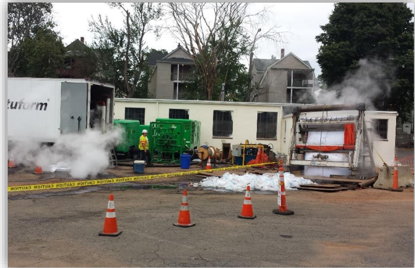
Installation of Cured-in-place-pipe (CIPP)
