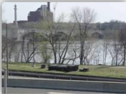
Discharge to River
