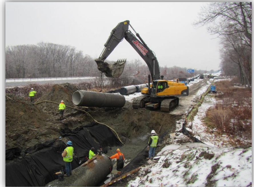
Installation of 48-inch PCCP along Route 57
