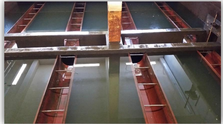
Existing FRP Backwash Troughs
