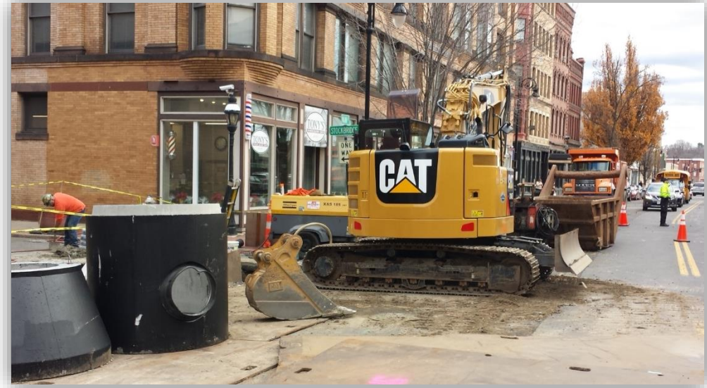
Replacement of 18-inch sewer within Stockbridge Street
