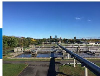
Wastewater Treatment Plant
