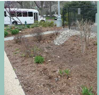
Figure 1: A bioretention cell absorbs runoff.
