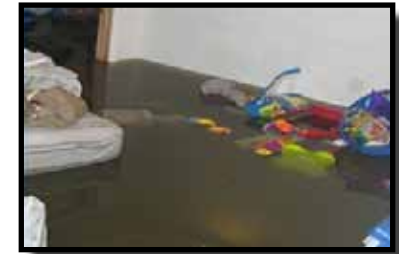
Avoid Sewer Backups in Your Home!
