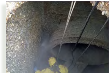
Cleaning MIS access structure prior to rehabilitation
