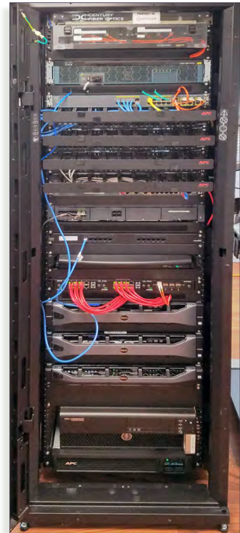
The new server rack at Provin Mountain Storage Tanks
