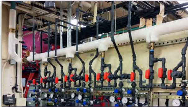
New Polymer Metering Pumps
