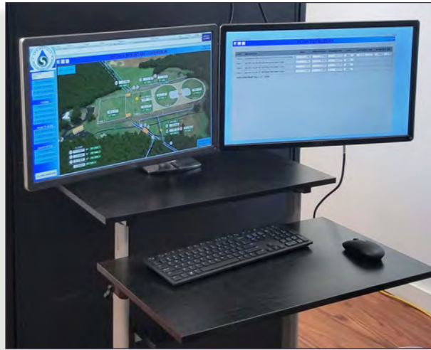
The new SCADA Station at Provin Mountain Storage Tanks
