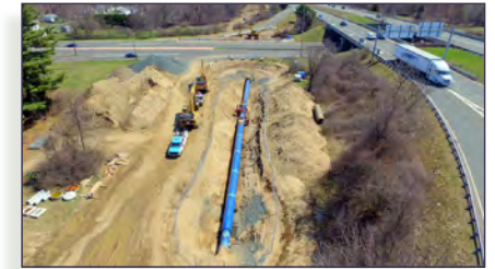
Aerial view of newly installed South Transmission Main along Route 57 in Agawam
