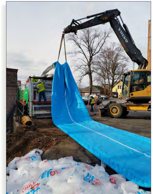
Liner for Main Intercepting Sewer before installation
