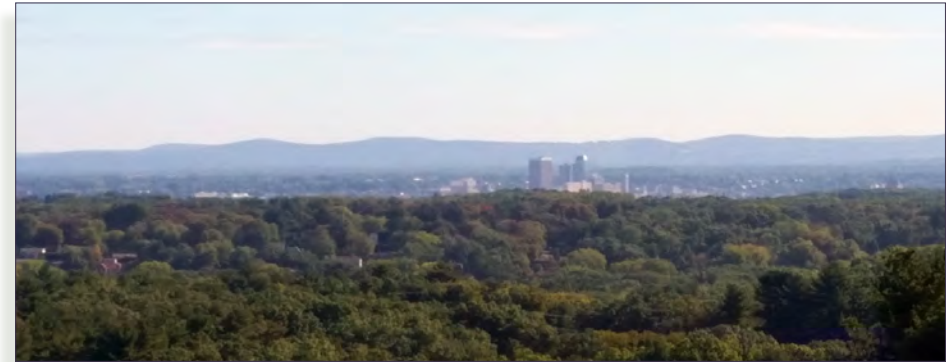
View of the City of Springfield from the top of Provin Mountain Storage Tanks in Agawam
