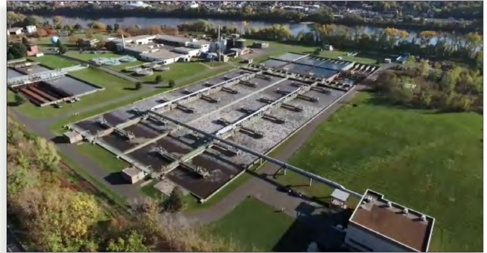
Springfield Regional Wastewater Treatment Plant
