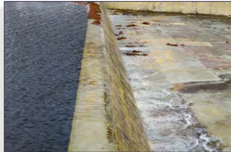
Cobble Mountain Dam Spillway
