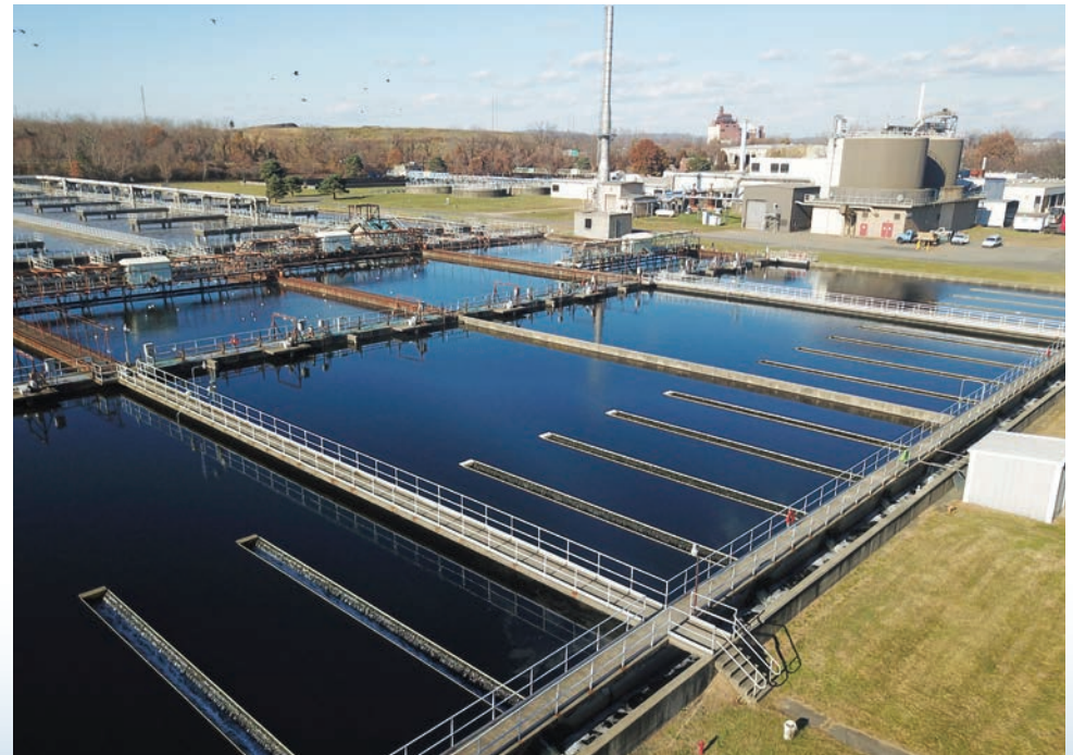
Top: The cast-in-place liner for the Main Interceptor Project is delivered for insertion, fall 2017. Bottom: The secondary clarifiers at the Springfield Regional Wastewater Treatment Facility.
