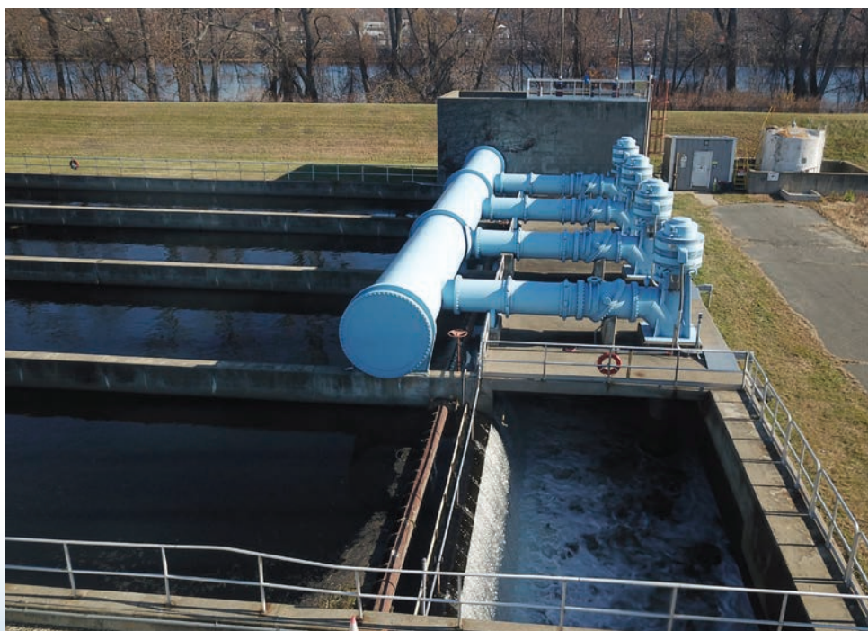
Above: As water exits the wastewater treatment process, it receives a final treatment of chlorine to eliminate remaining bacteria, and then flows into the Connecticut River.
