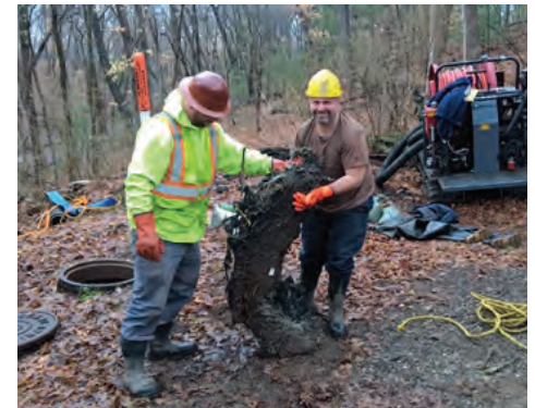
Above: Grit, oils, grease, and other debris removed from the South Branch Sewer main in the Sixteen Acres area of Springfield, April 2017.
