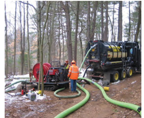
Above: High-pressure cleaning of a sewer line through a manhole (seen at left in the picture) in the Sixteen Acres area of Springfield, April 2017.
