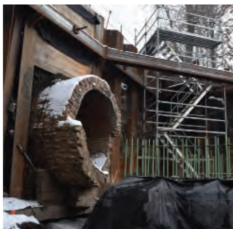
Above: The headwall of a combined sewer overflow outfall is reinforced as part of the Main Interceptor Sewer and Combined Sewer Overflow Outfall Improvements Project.
