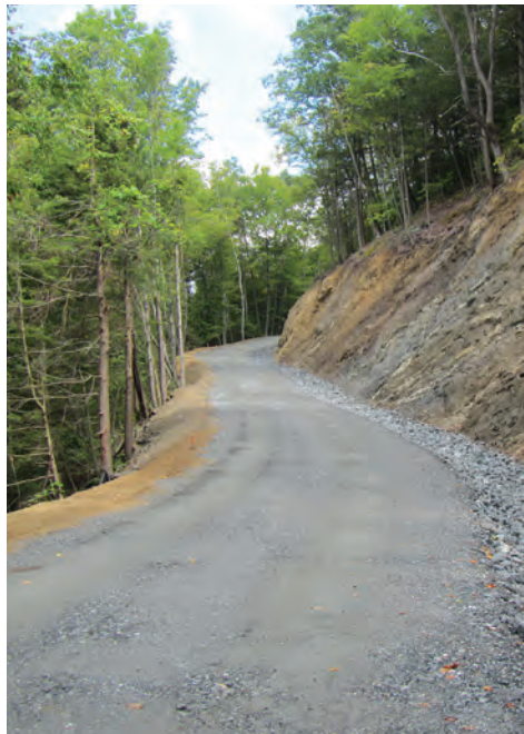
Above: The Intake Dam Road was widened to allow for better maintenance and emergency access.
