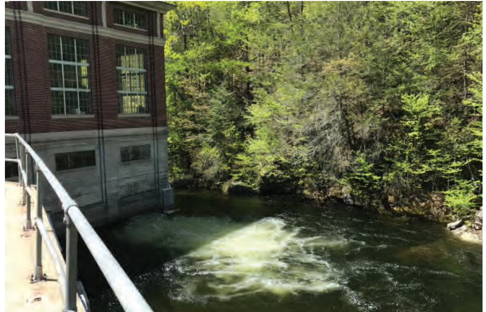
Above: The Cobble Mountain Hydro-Energy Power Plant, located in Granville.
