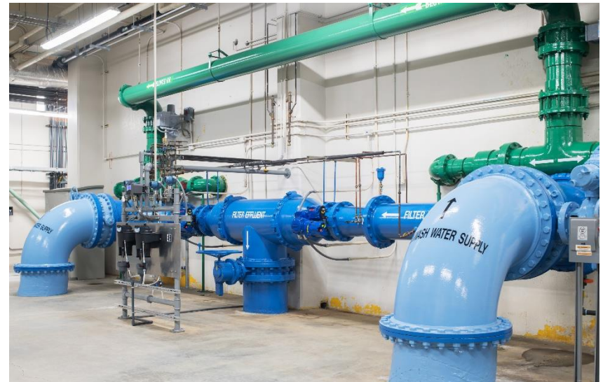
Pipe gallery at West Parish Filters.
