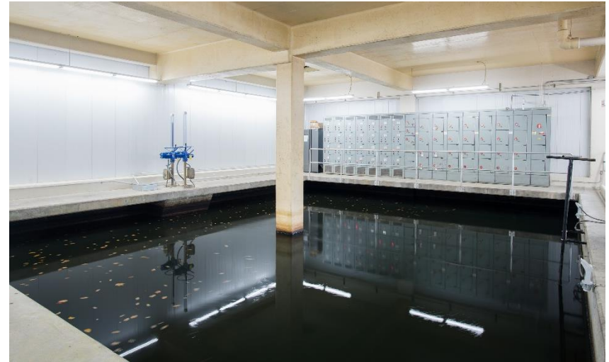
Rapid Sands Filter at West Parish Filters.
