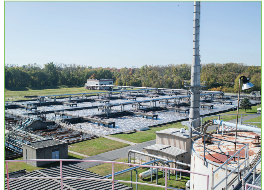
Above: The aeration basins at the Springfield Regional Wastewater Treatment Facility.
