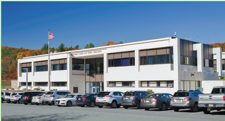
Above: The West Parish Filters Water Treatment Plant in Westfield.
