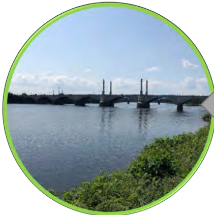
Discharge to CT River
