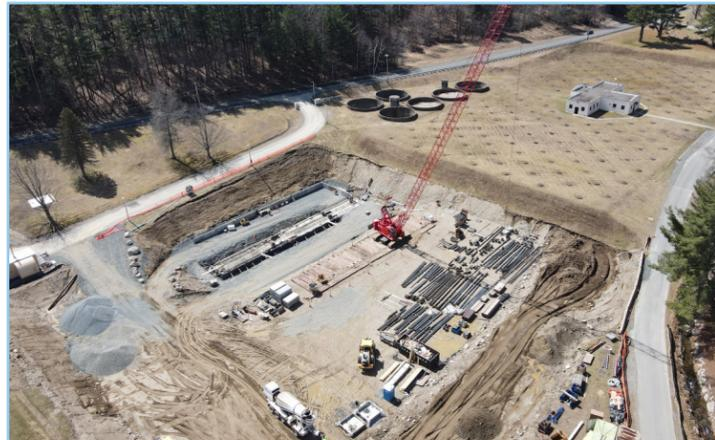
In 2021 the Commission broke ground on a new era of drinking water treatment at West Parish Filters. Phase 1 construction of the new water treatment plant is currently underway, with construction of the new Clearwell and Backwash Pump Station Replacement Project. Original 1909 slow sand filters were demolished to make way for a new filtered water clearwell.
