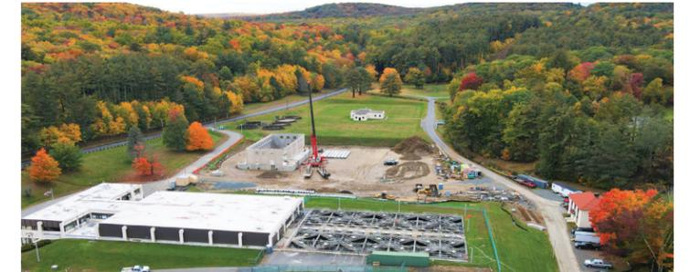
Phase 1 Construction: The new clearwell under construction at West Parish Filters Water Treatment Plant in October 2022.
