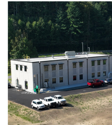
The new Backwash Facility at West Parish Filters was completed in fall 2023.
