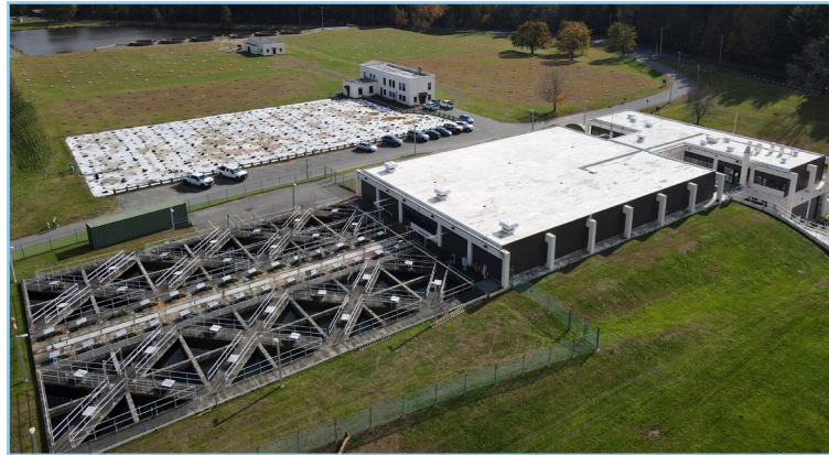
West Parish Filters Drinking Water Treatment Plant in Westfield, MA was originally built in 1909 and last modernized in 1974.
