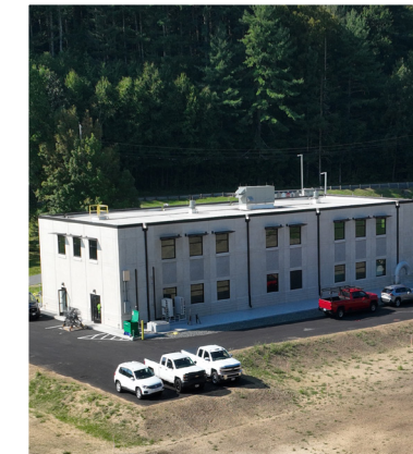
The new Backwash Facility at West Parish Filters was completed in fall 2023.
